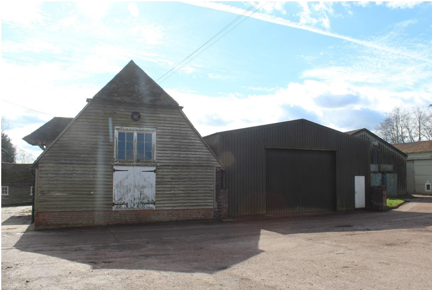
Plate 19: View of the northern end of the threshing barn with the modern barn to the west. (Facing S).
