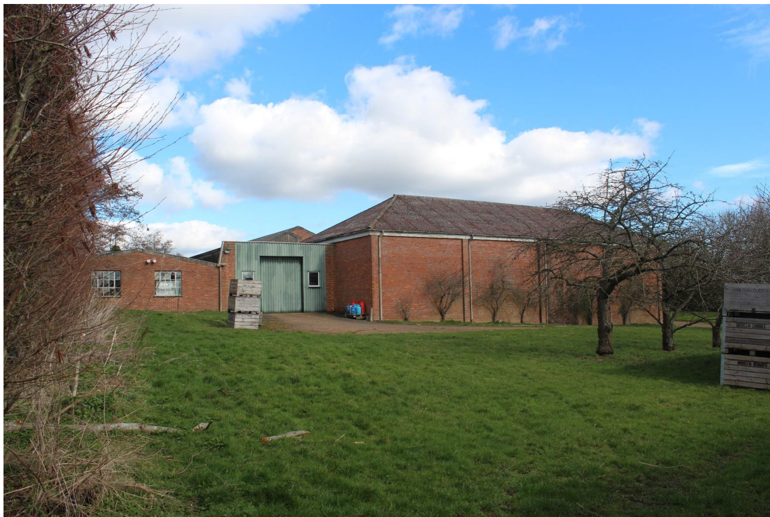
Plate 23: View of southern end of the modern buildings from the current south west corner of the PDA (Facing NNE).
