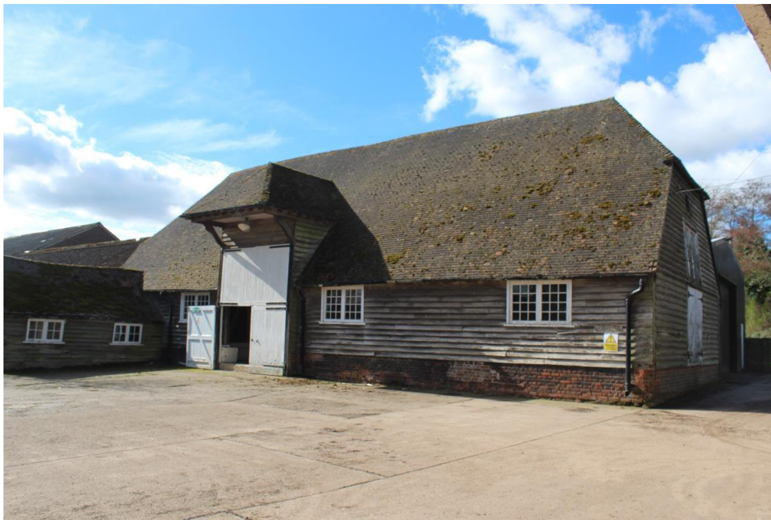
Plate 11: View across PDA towards the threshing barn and part of the eastern extension (facing SW).
