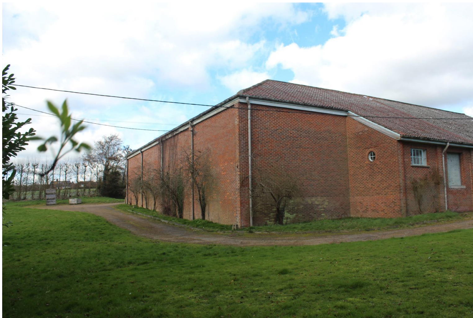
Plate 22: View of southern end of the modern building that faces the road (Facing NW).
