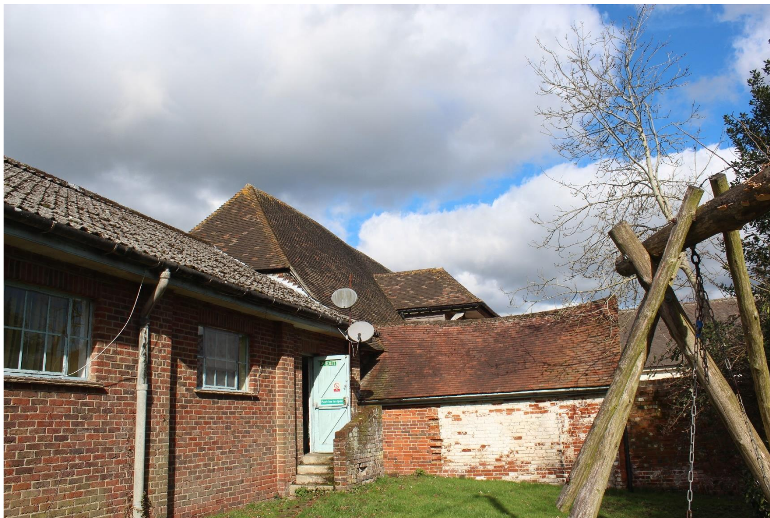
Plate 21: View of the rear of the threshing barns eastern building with the modern building (Facing NW).
