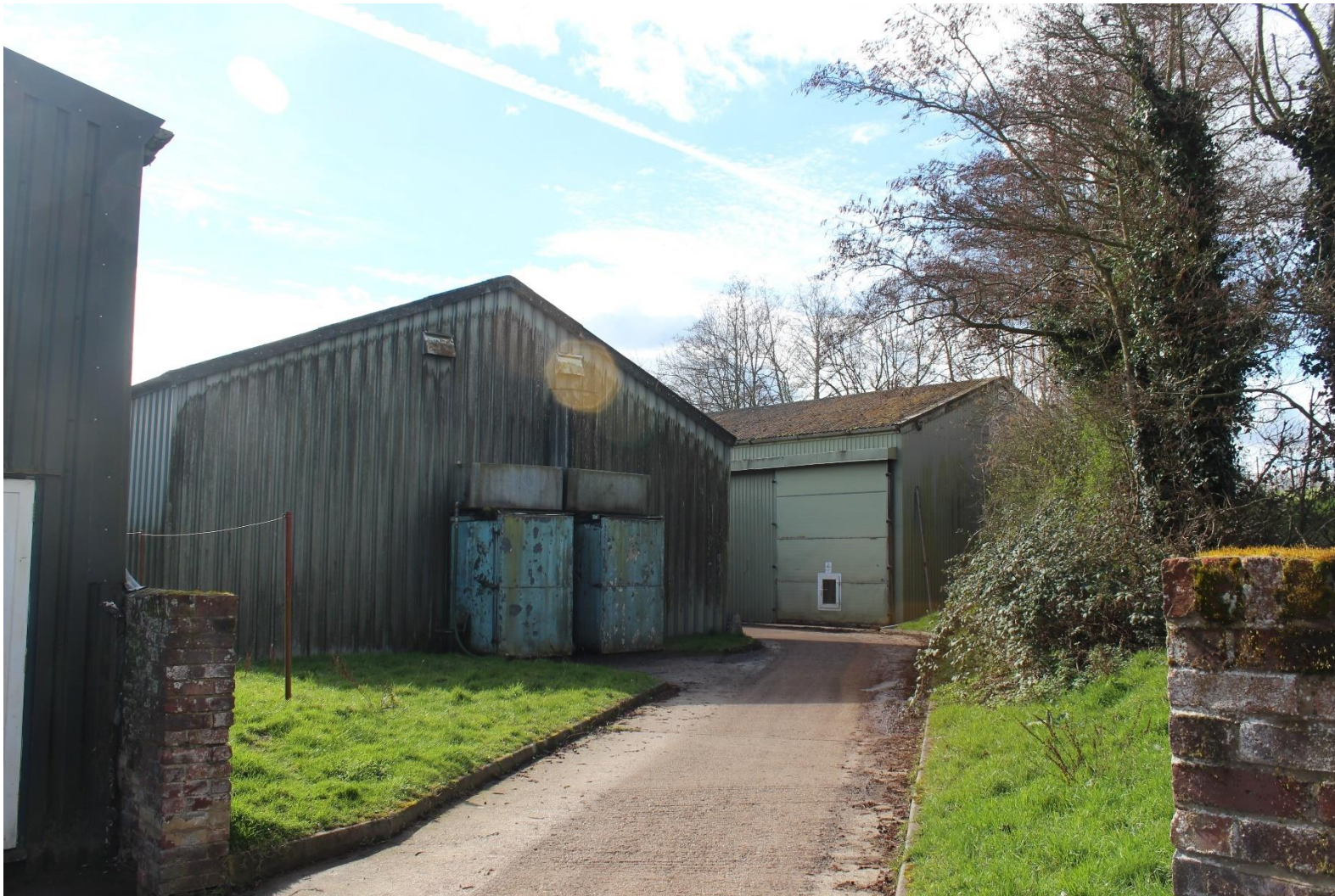
Plate 17: View of the modern buildings within the PDA at the western side (Facing SSW).
