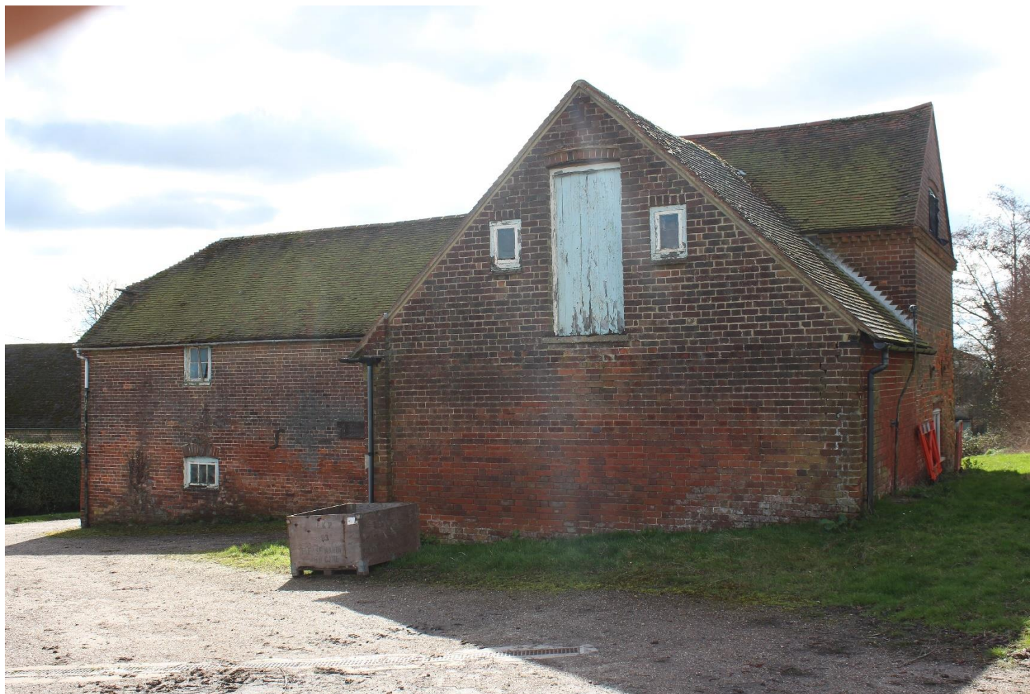
Plate 16: View at the northern end of the PDA towards the rear of the oast (Facing S).
