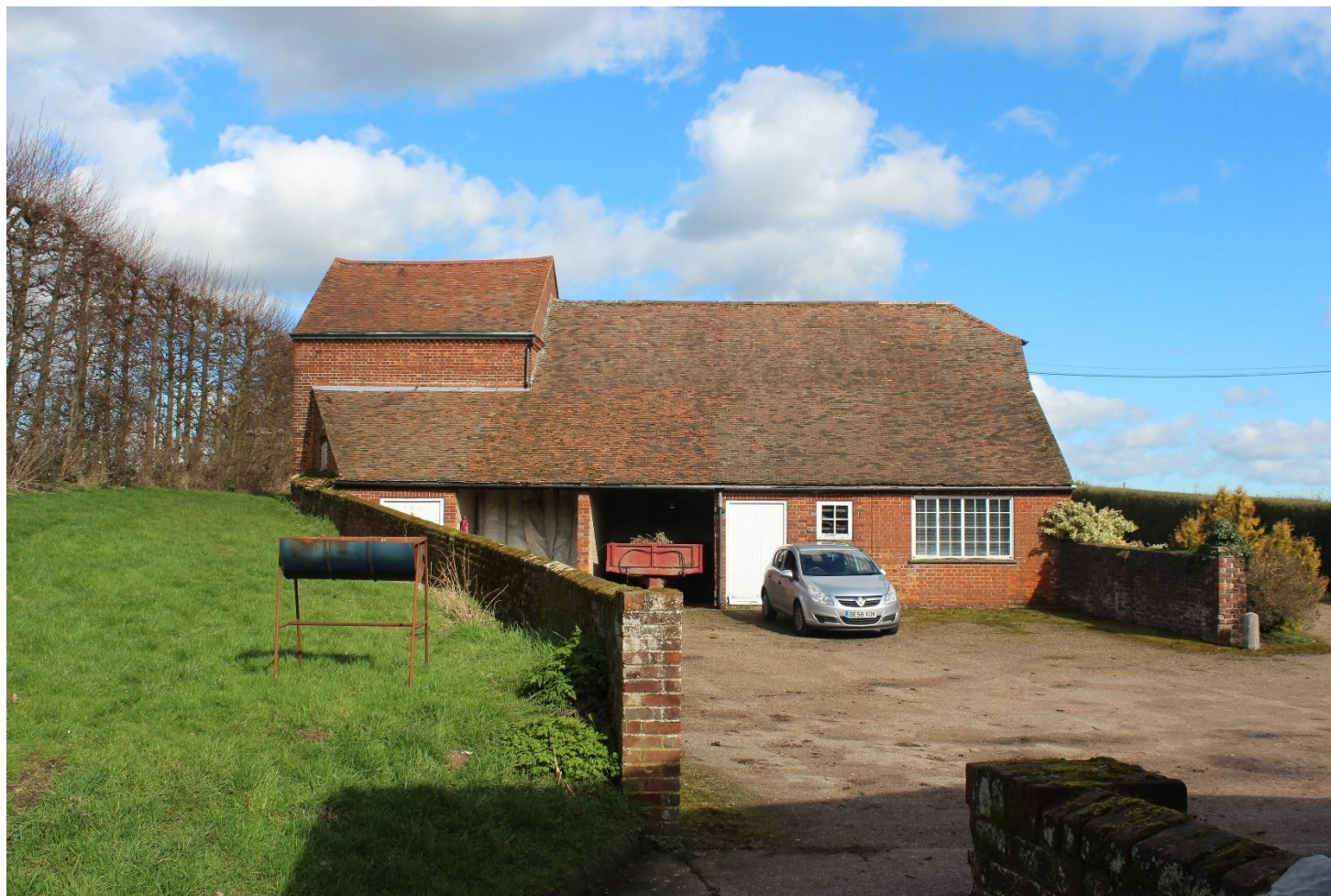
Plate 13: View of the oast at the northern end of the PDA (Facing N).
