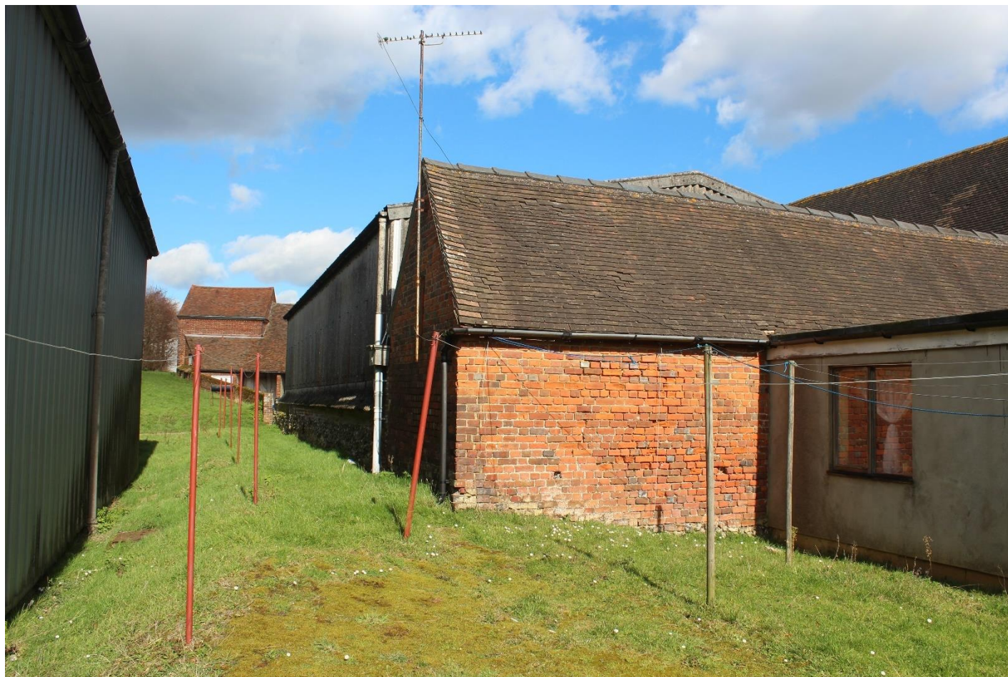
Plate 18: View of the rear of the card shed extension to the threshing barn. (Facing N).
